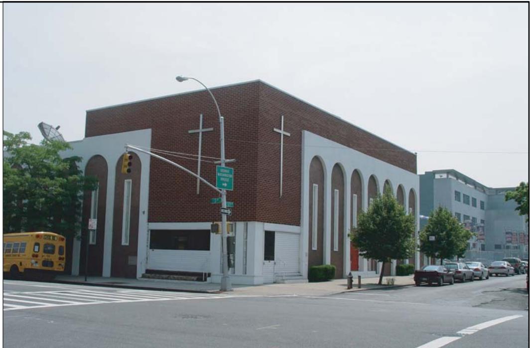
Viewpoint 08 - View looking east at E 127th Street & Third Avenue
