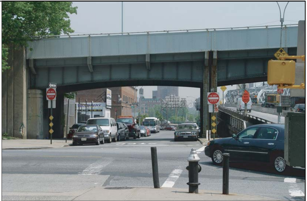
Viewpoint 29 - View of First Avenue looking north towards Willis Avenue Bridge
